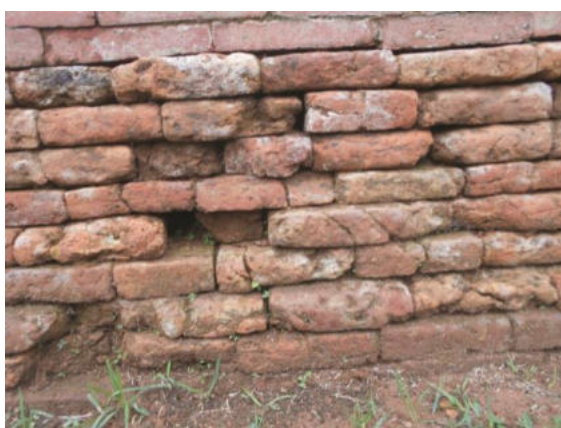
Plate 56.7: Mixed bond brick setting, temple wall of ShalbanVihara Photo : Author.
