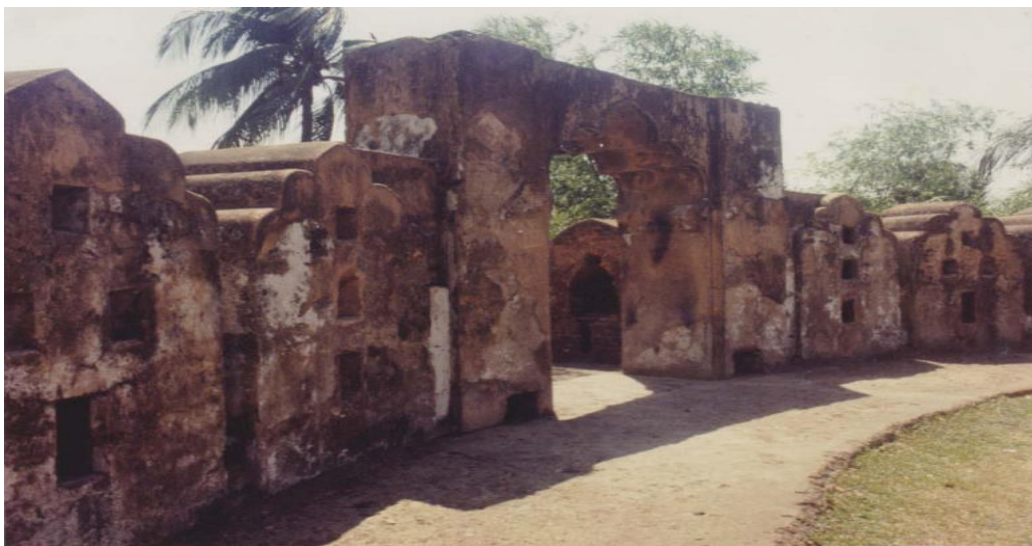
Plate 53.10: Surrounding wall crowned with big merlons, Sonakanda River Fort.
