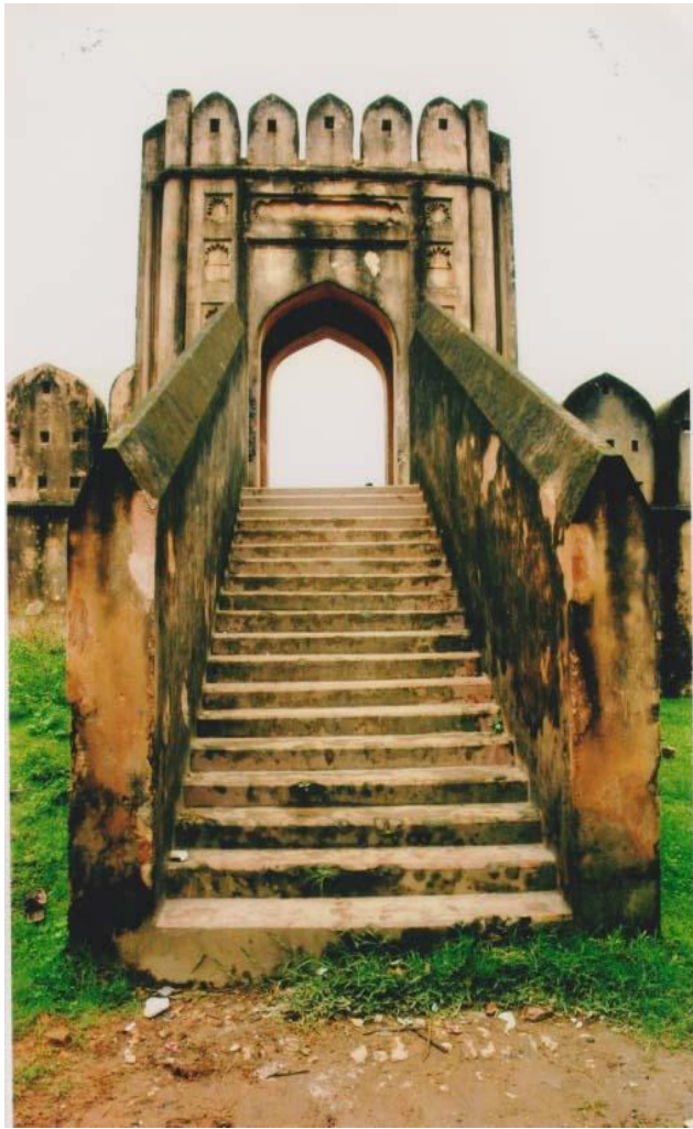
Plate 53.3: Gateway of Hajiganj River Fort, Narayanganj, view from outside.
