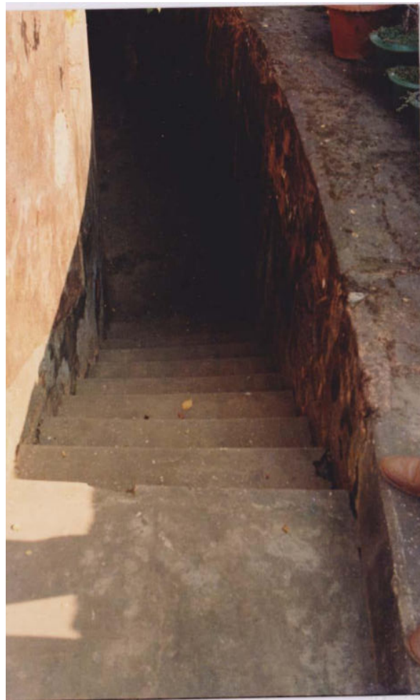
Plate 53.16: Staircase leading towards Basement Chamber, Idrakpur River Fort.
