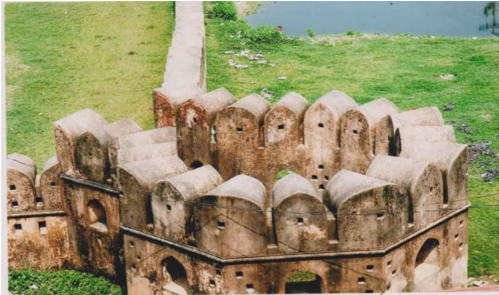
Plate 53.6: Corner Bastion, Hajiganj River Fort, Narayanganj.
