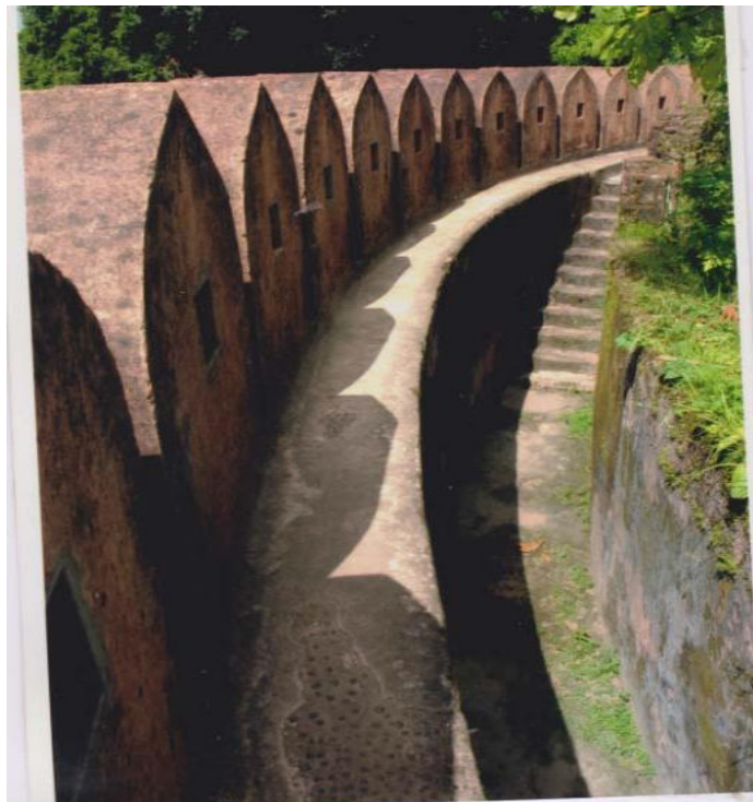
Plate 53.7: Rampart Pathway, Hajiganj River Fort, Narayanganj.
