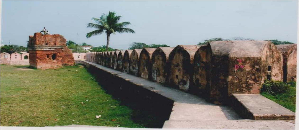
Plate 53.4: Parapet wall with loopholes, Hajiganj River Fort, Narayanganj.
