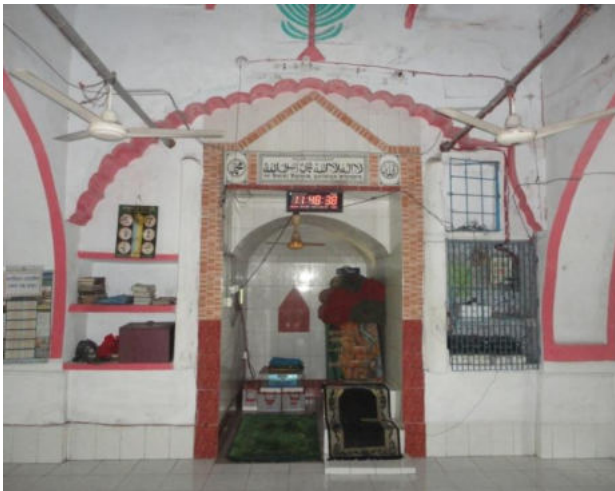
Plate 11.35b: Original feature of the central Mihrab was totally renovated and the alcove was pushed inside thus a wide projection was created. The semicircular arch was rebuilt and lost the scale. The cusped arched border bordering the alcove was also renovated and shelves and storage were created.
