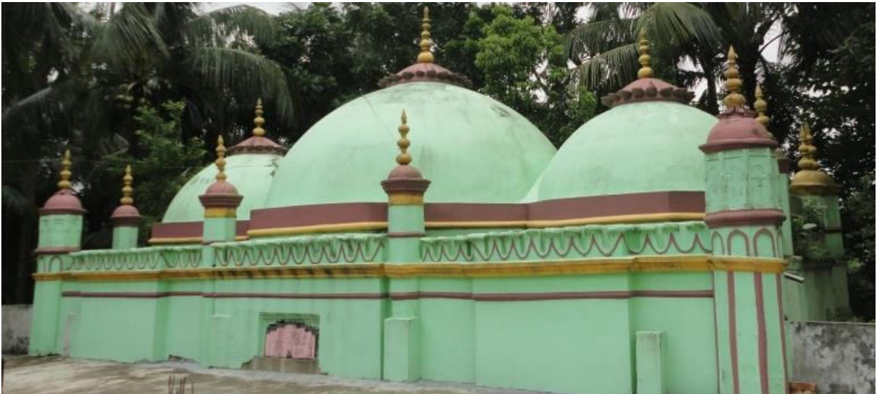
Plate 11.27: Present view of the original Matubi Mosque.
