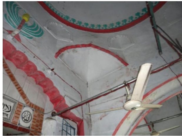
Plate 11.38a: Phase of transition (semi vaults and shallow arched alcoves with cusped design to place the dome on a square central bay of the prayer hall).
