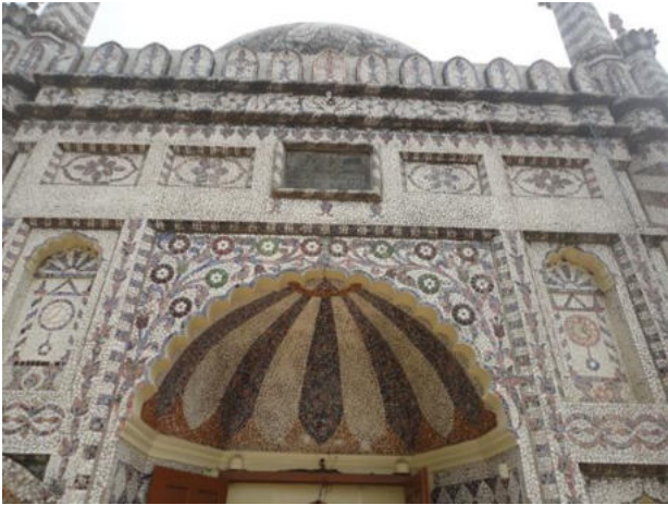
Plate 11.7: Semi Vault of central arched entrance.
