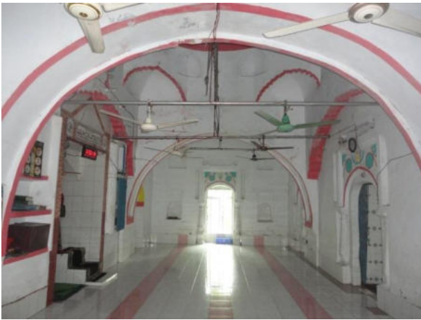
Plate 11.37: Semicircular Lateral arch dividing the prayer hall into three unequal bays.
