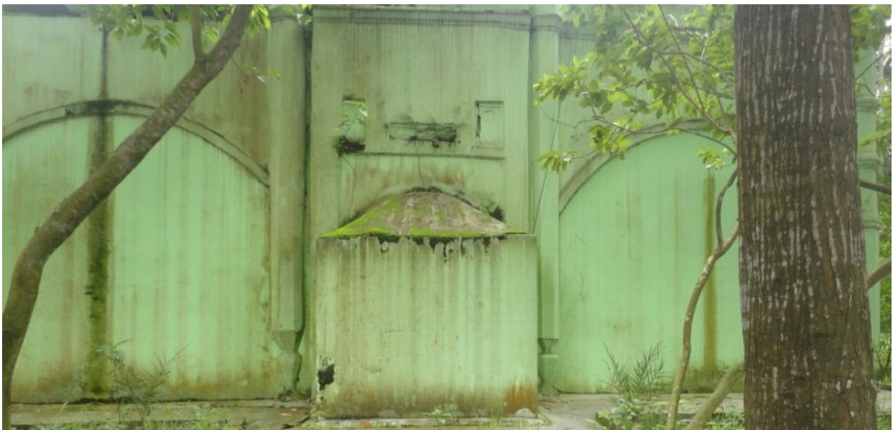
Plate 11.35d: Distorted tri-partition of the Qibla wall from outside, the outline of flanking mihrabs are slightly wider than the central mihrab area. The central mihrab area is projected and flanked by two engaged turrets with Kalasa base. The flanking mihrab or bay is outlined with an arched design.
