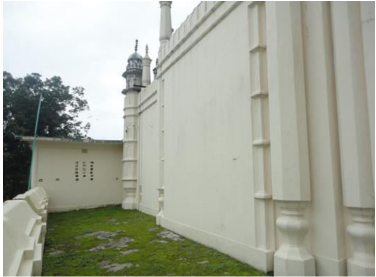
Plate 11.14: Qibla wall of the mosque highlighted with nook shaft and side turrets with Kalasa base.
