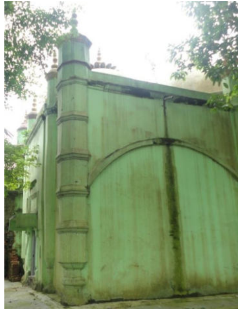
Plate 11.33: Octagonal corner tower with Kalasa base and moulding at intervals reminds the Mughal style. Due to restoration features of alcoves are missing.
