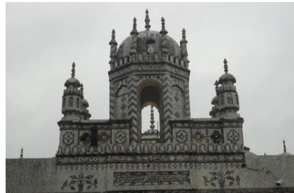
Plate 11.4: Kiosk and Balcony of eastern gateway.
