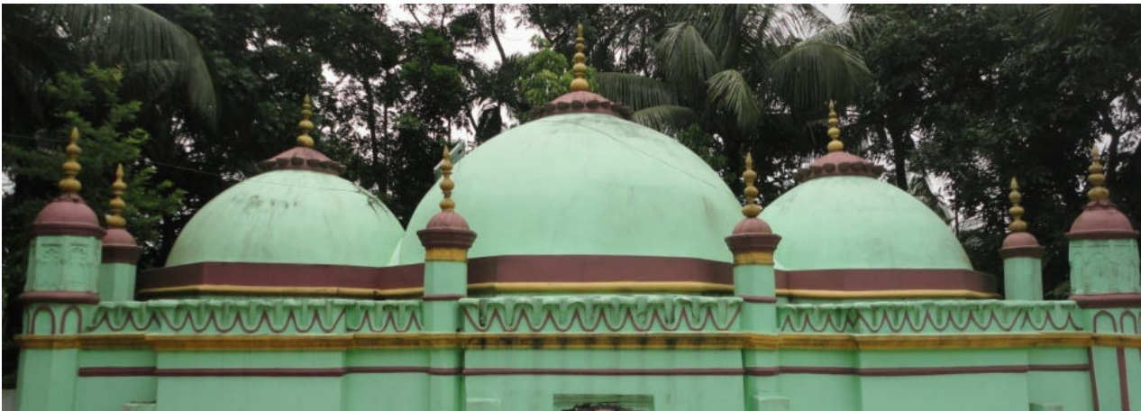
Plate 11.40: Three wide domes (Mughal proto type) resting on octagonal shoulders with abstract lotus design and kalasa motifs. The domes are further highlighted by corner towers and engaged turrets thus creating a skyline of the mosque.
