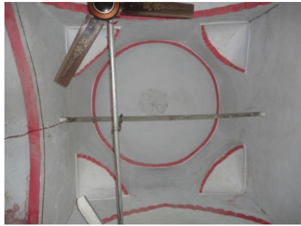
Plate 11.39: Phase of transition for the side domes achieved through solid blocks and archways supported by northern and southern wall and lateral arches of both side bays.
