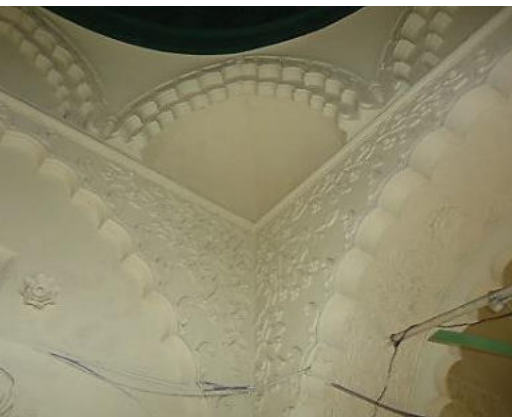
Plate 11.17: Semi vault constructed to set dome on the central bay.
