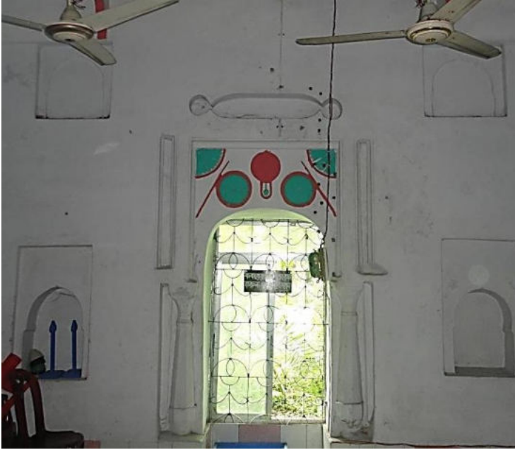
Plate 11.32: South Side entrance of the mosque semicircular arch rests on balustrade type of columns outlined with a rectangular recessed border. Flanked with two arched alcoves. On top a slim rectangular panel (Mughal style) can be seen which is again flanked with arched recess. Spandrel depicts the remnants of Fan designs these were probably distorted during restoration work.
