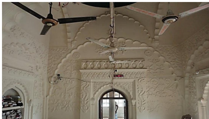
Plate 11.18: Springing cusped arches parallel to Qibla wall and arched recess on north wall with semi vaults accommodated a dome upon a rectangular space on the north bay.
