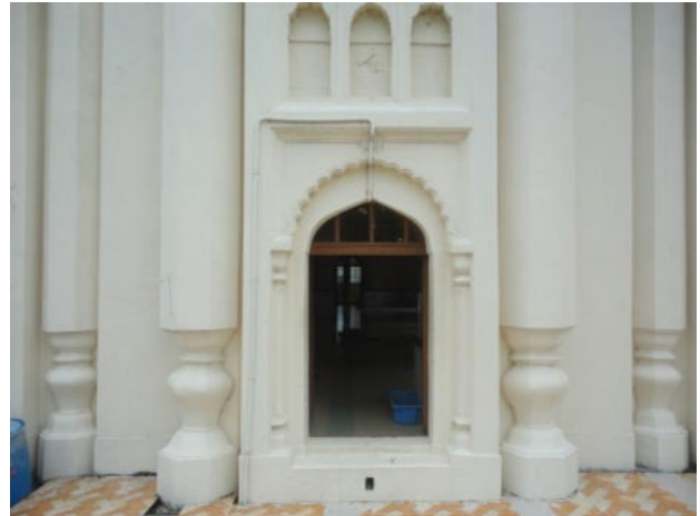
Plate 11.8: Single arched opening on the south side.
