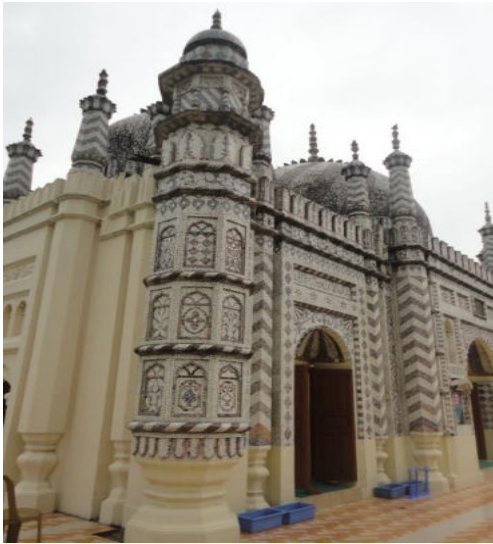
Plate 11.13: Octagonal Corner tower with kalasa base, blind kiosks cupola and finial of southeast corner.
